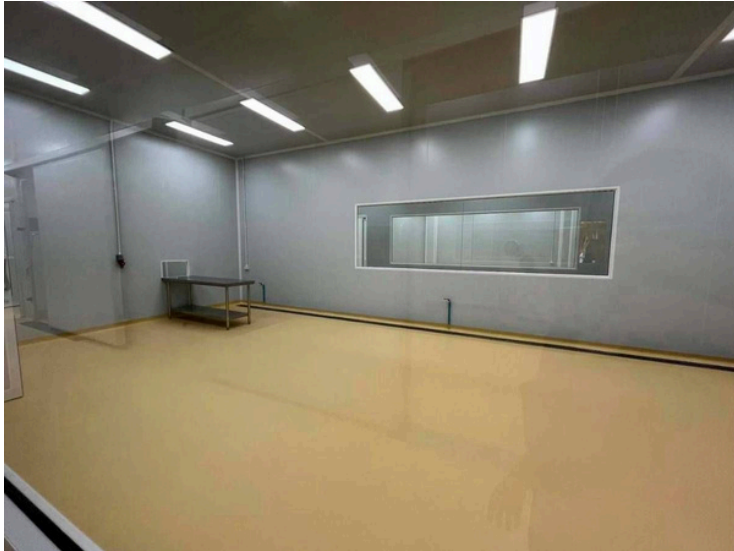
Renovation & Built-In Services
